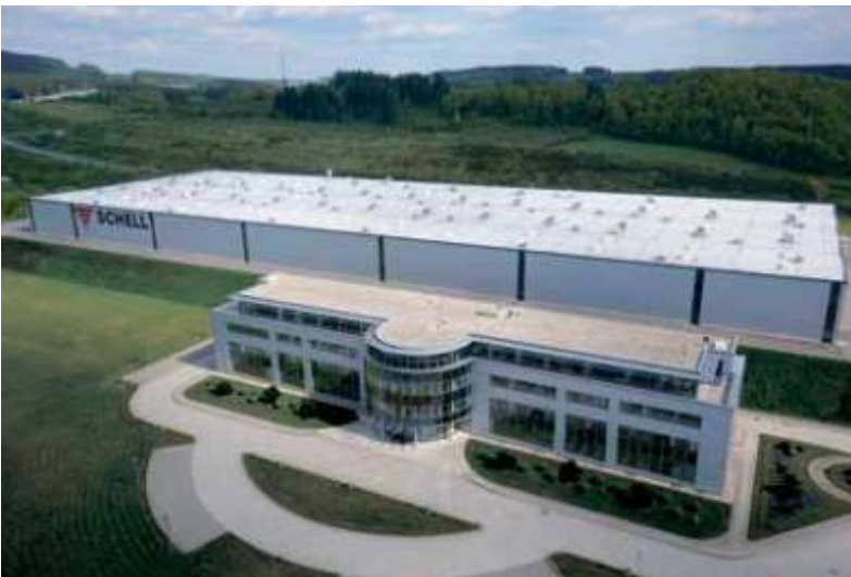
Plant 1 Production with administration and training centre
