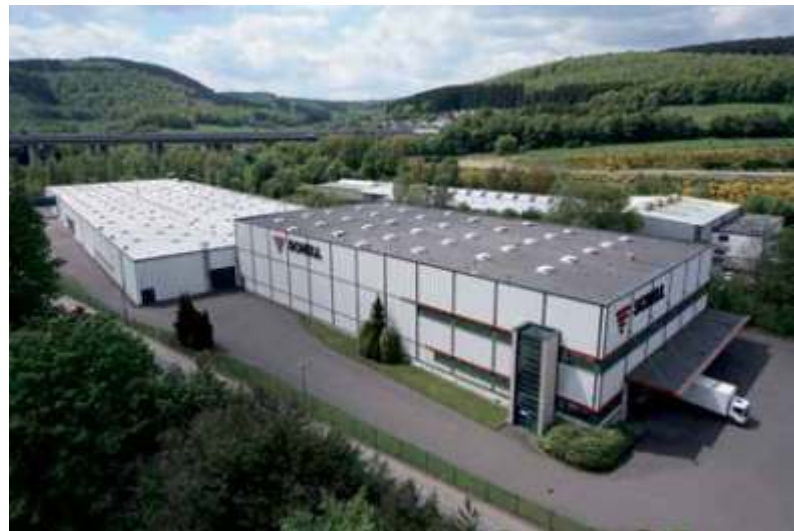
Plant 2 Production with logistics centre
