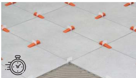
5. After Levelling Process leave it for 8-10 hrs.
