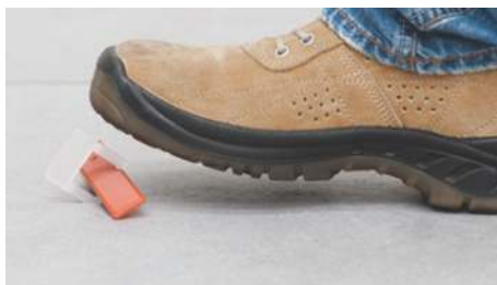
6. Remove Wedges ones it Dry
