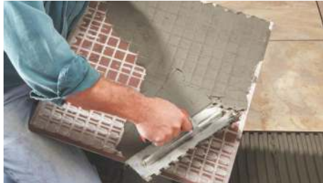
2. Cement laying on Tile
