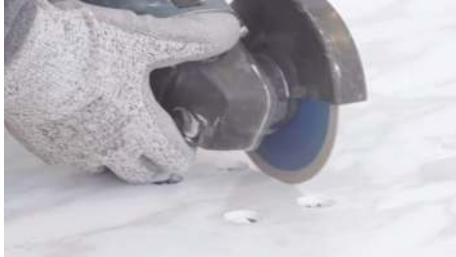
2. Cut with Diamond Blade Angle Grinder
